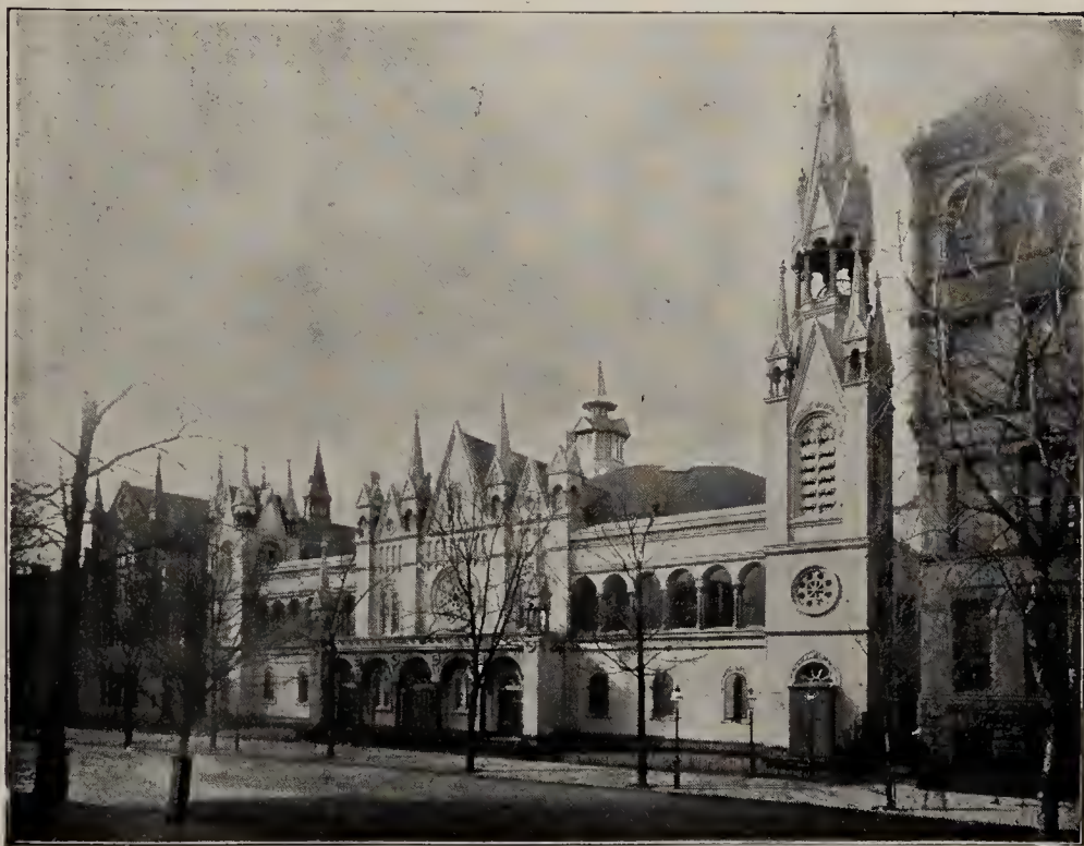
CENTRAL CONGREGATIONAL CHURCH
